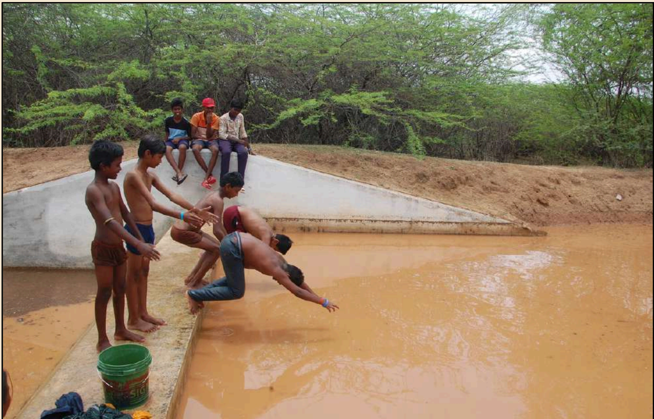
Check-dam constructed by the AF-EC impounds water at Yerraborepalli village in Setturu Mandal of Anantapur district.
